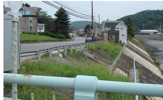
View from Hickory Street Bridge.
